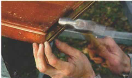
The bottom gets a hook strip. After the bottom of the door is sealed, a hook strip is nailed into the rabbet.
